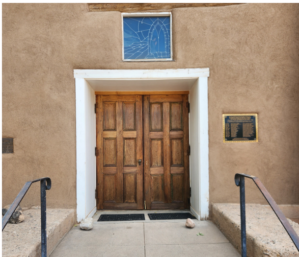
The Old Church doors were stained as part of the exterior replastering project.
