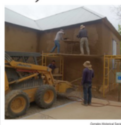
Working on the exterior of the Old Church
