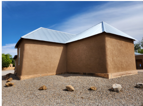
A view of the completed replastering
