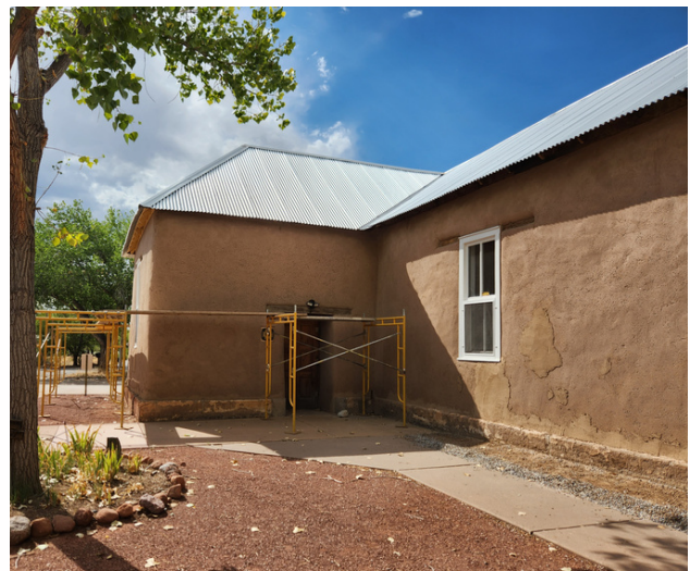
The South Transept replastering
