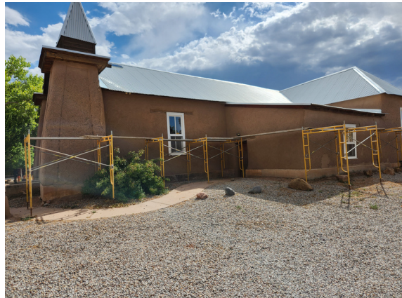
Exterior replastering of Old Church
